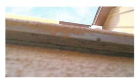
This gap needs to be protected with screening or sealed off with caulking, fire resistive foam, mortar, or similar product.
