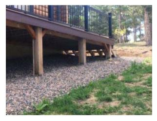
require significant maintenance to keep it from drying out and splitting. The dry and split wood is very susceptible to capturing embers and igniting.
